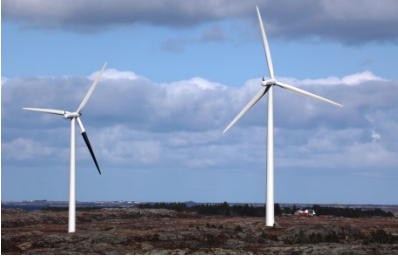
The research project conducted at Smøla wind farm using contrast paint and UV light to increase visibility was concluded in 2016.
