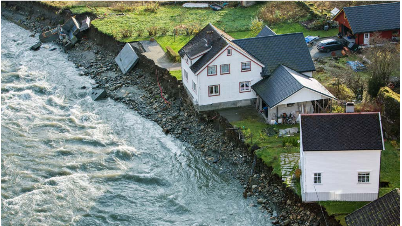
Extreme weather has major consequences. Pictured here from Flåm in Norway where heavy rainfall made the river overflow its banks, causing severe damage. Photo: Tore Meek/NTB scanpix.
